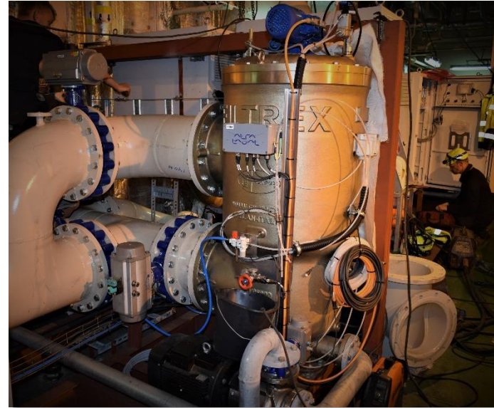
Vessel Installation Works
