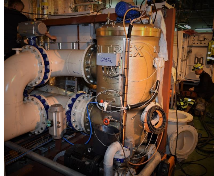
Vessel Installation Works
